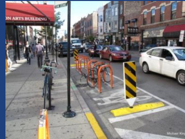
On-Street Bike Corral in Chicago, IL Credit: Chicago Complete Streets
