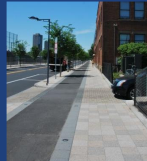
Vassar Street Protected Bike Lane Cambridge, MA
