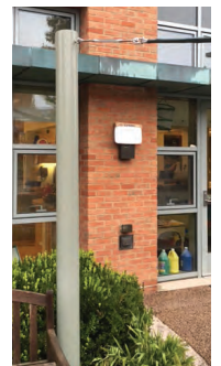
Canopy corner mounted to pole structure
