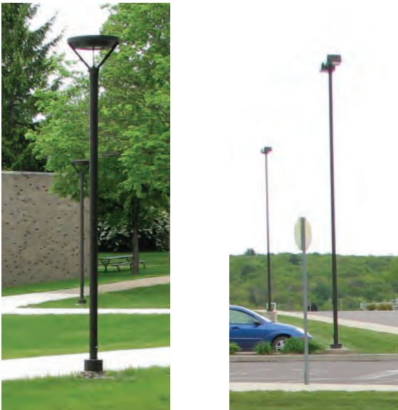
Campus standard LED Largent light fixtures
