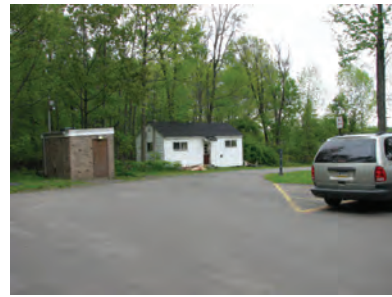
Demolish Inspector's House
