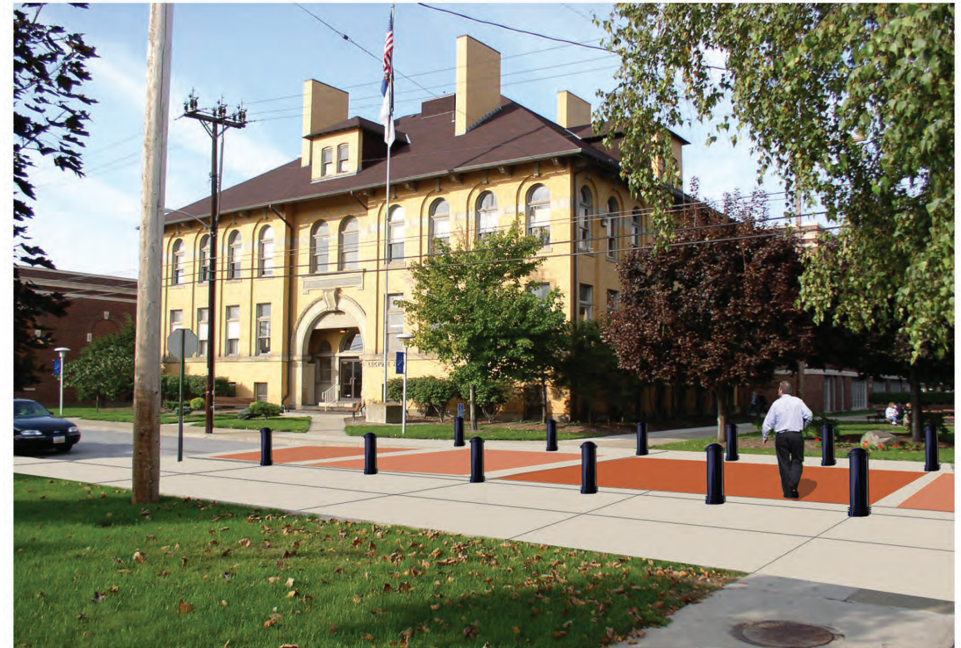
Shenango Avenue at the campus mall after lane reduction and paver installation
