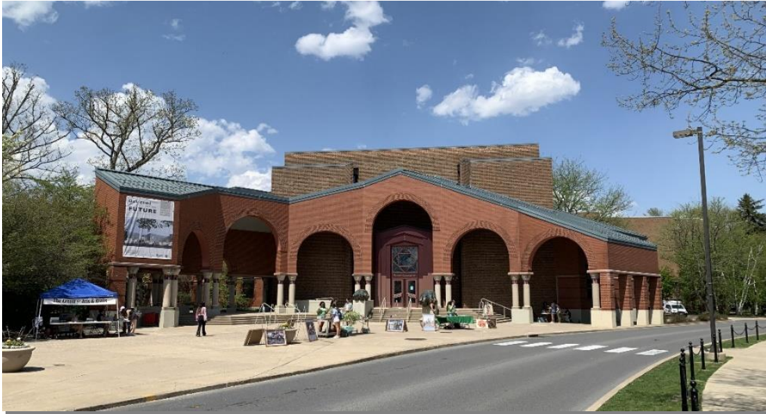
Photo above: Front view of existing building
