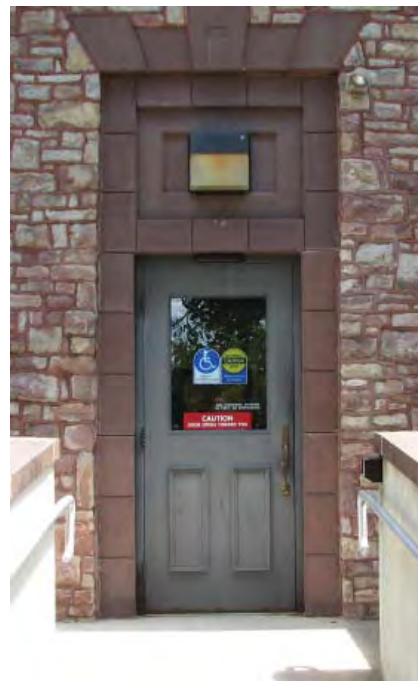
"Utility style" fixture to be avoided
