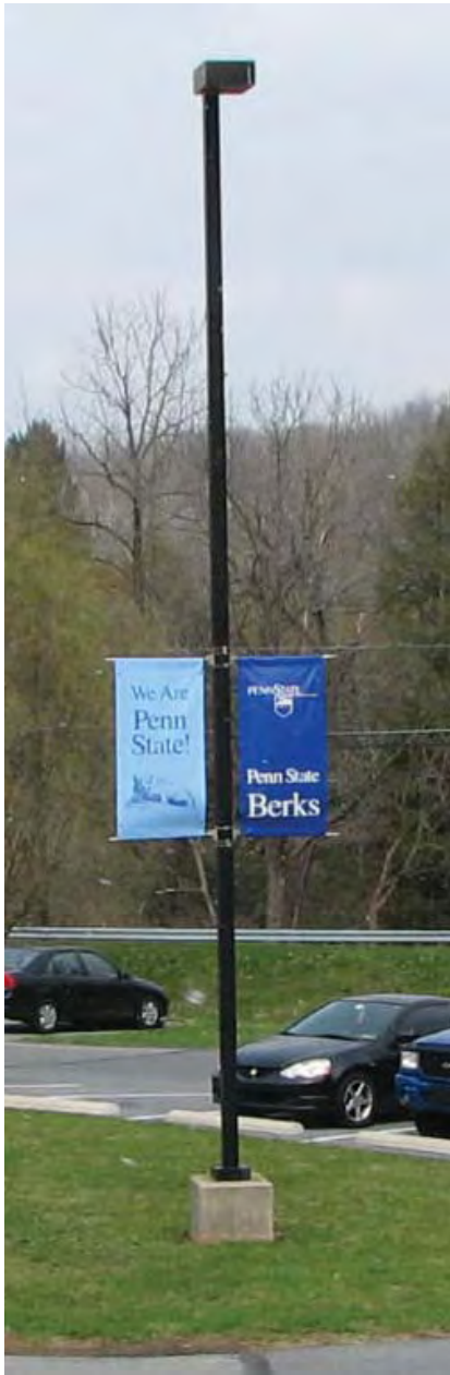
Typical Parking Lot/Roadway Light
