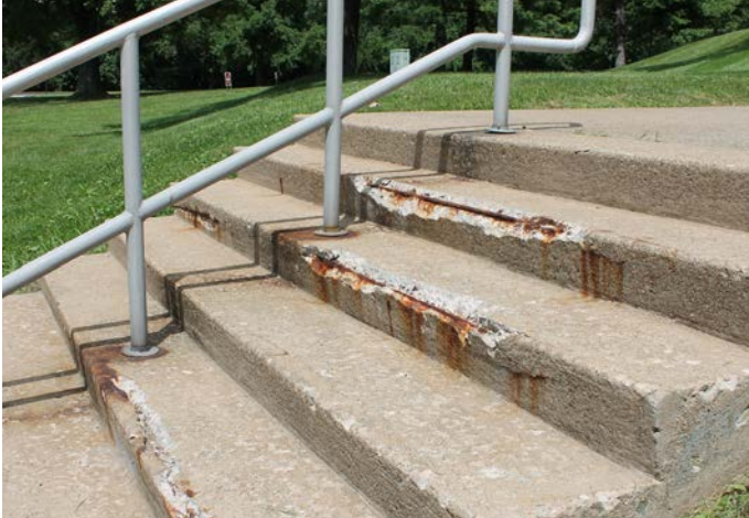
Exposed rebar
