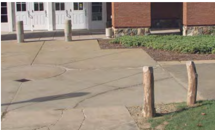
Existing site bollards
