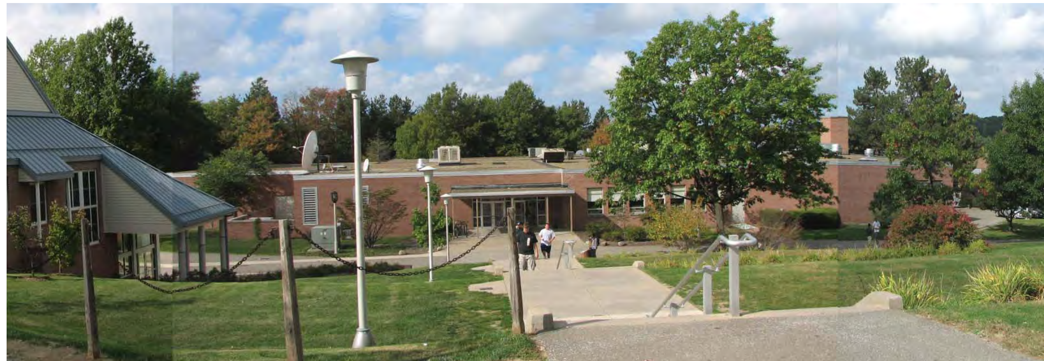
View of existing roof
