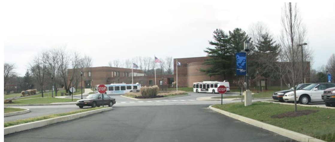
Existing view into Brandywine campus from entrance drive
