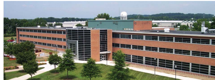
Addition at main entrance to Olmsted Building - Harrisburg
