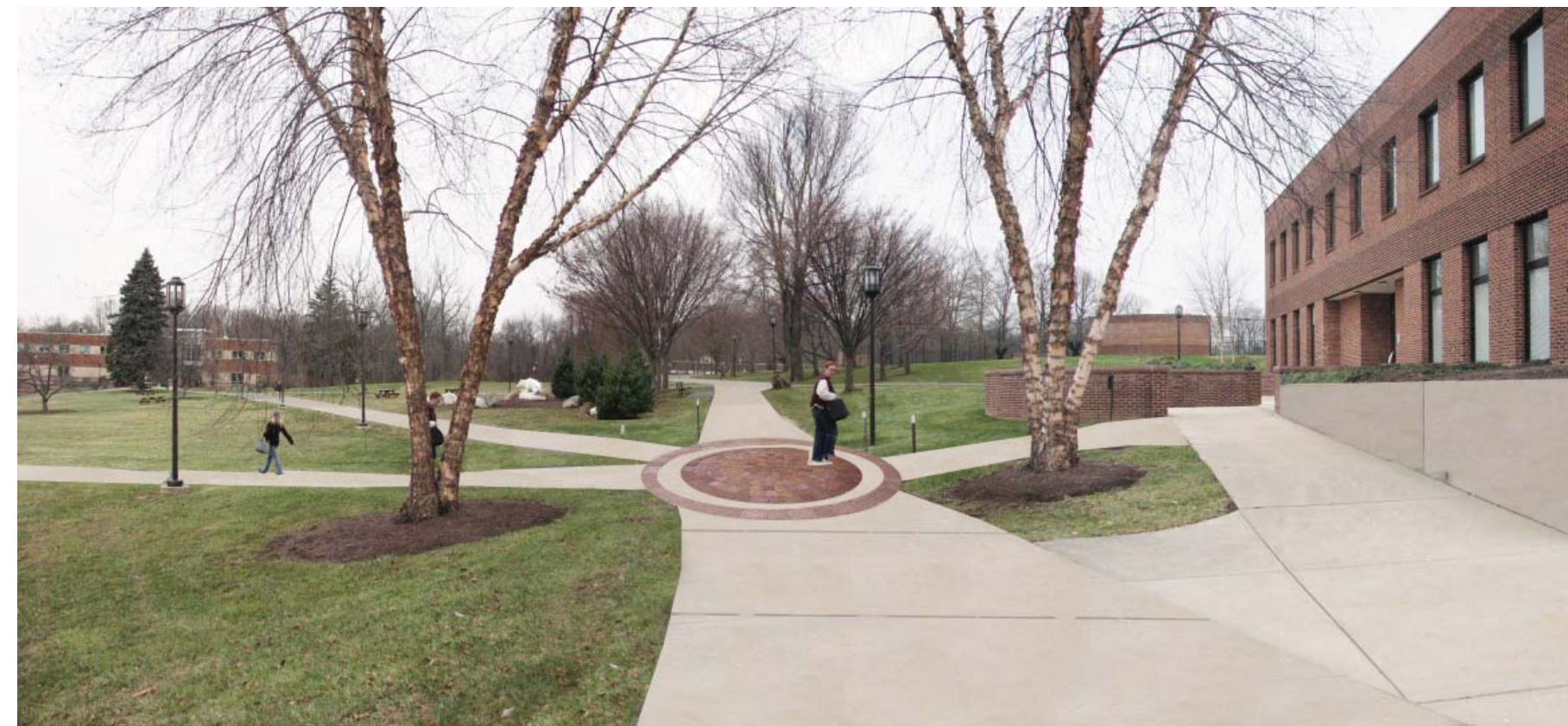
New concrete walks with brick paver nodes
