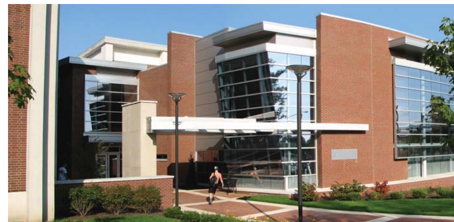
Rec Hall addition along Atherton Street - University Park
