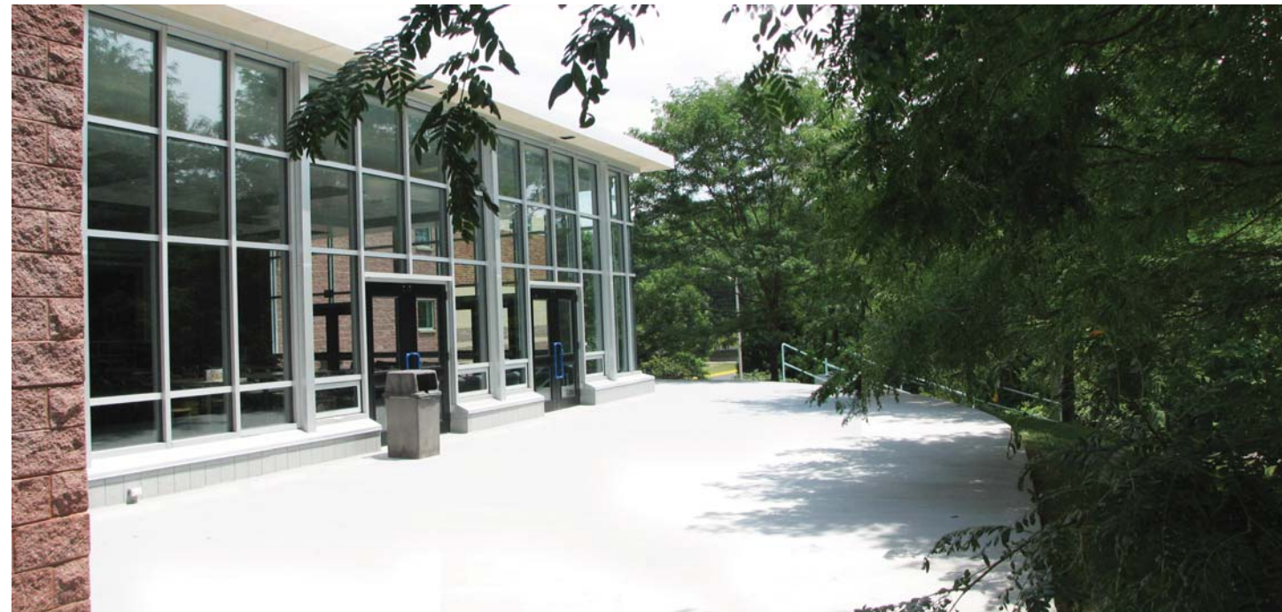
Existing Tomezsko Classroom Building back patio
