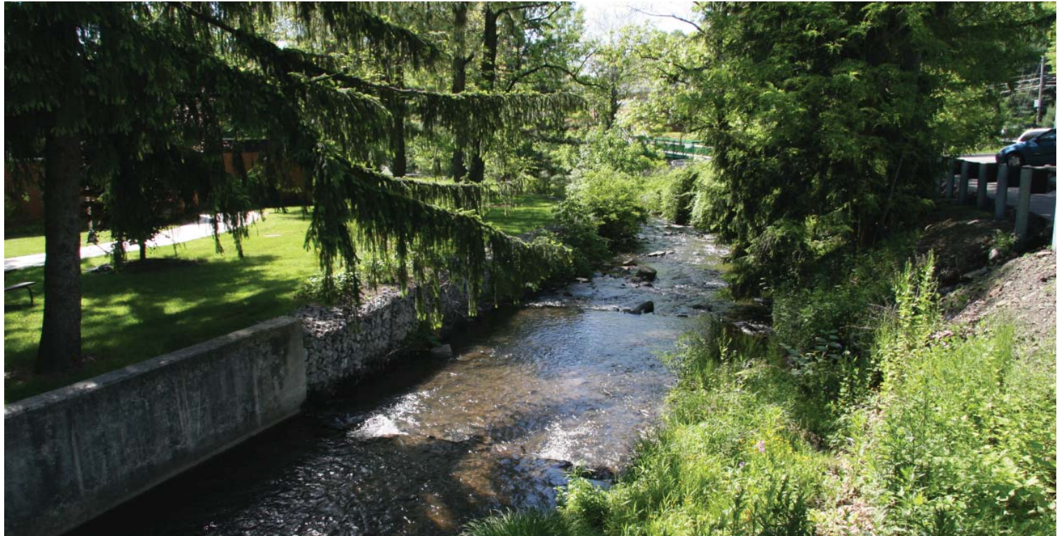
Existing engineered stream edge
