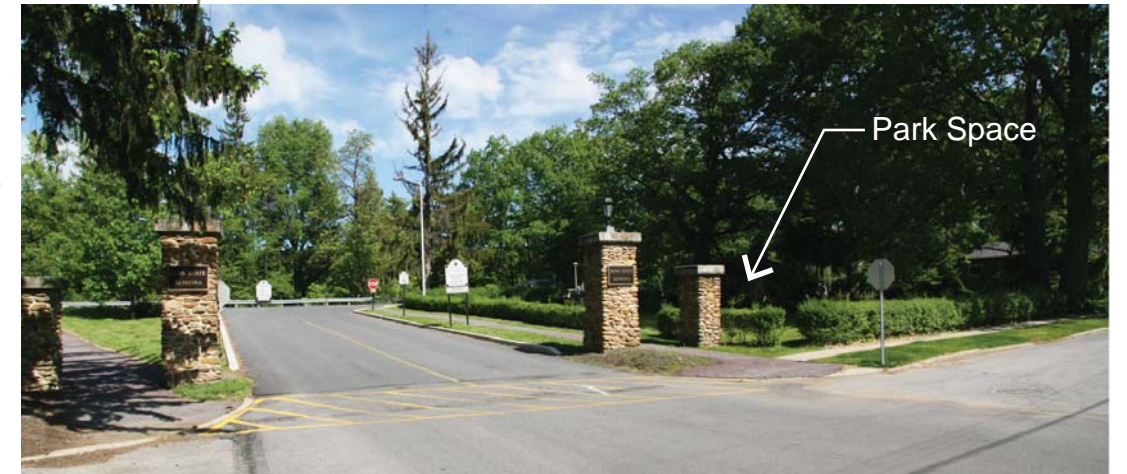
Existing campus entrance at Ivyside Drive
