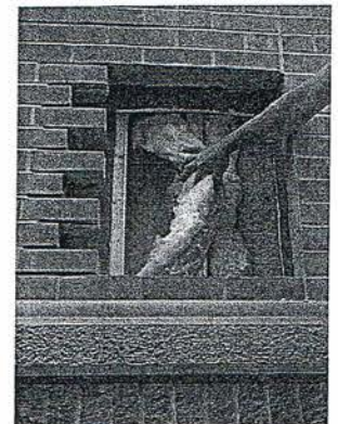
Interior Vapor Barrier, Plywood, and Gypsum Board
