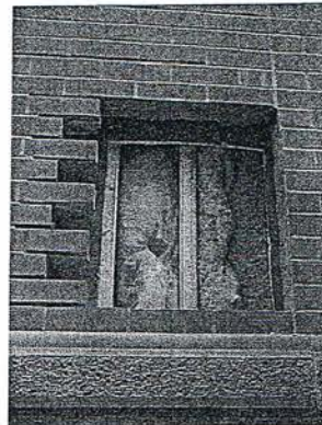
Interior Metal Frame Wall and Fiber Insulation
