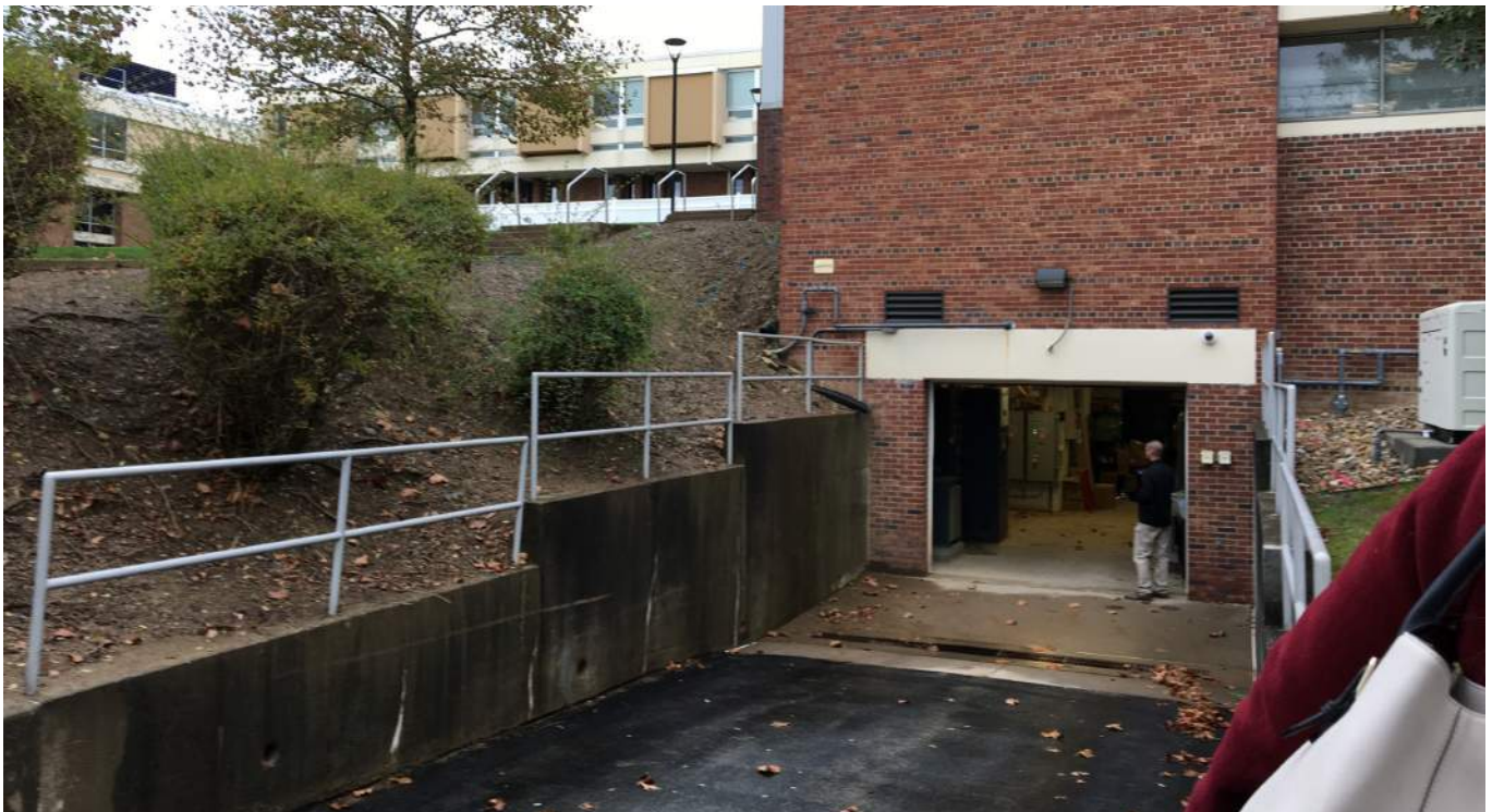
Existing Loading Dock
