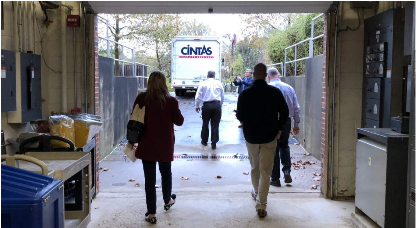
Existing Sub-Basement Level
