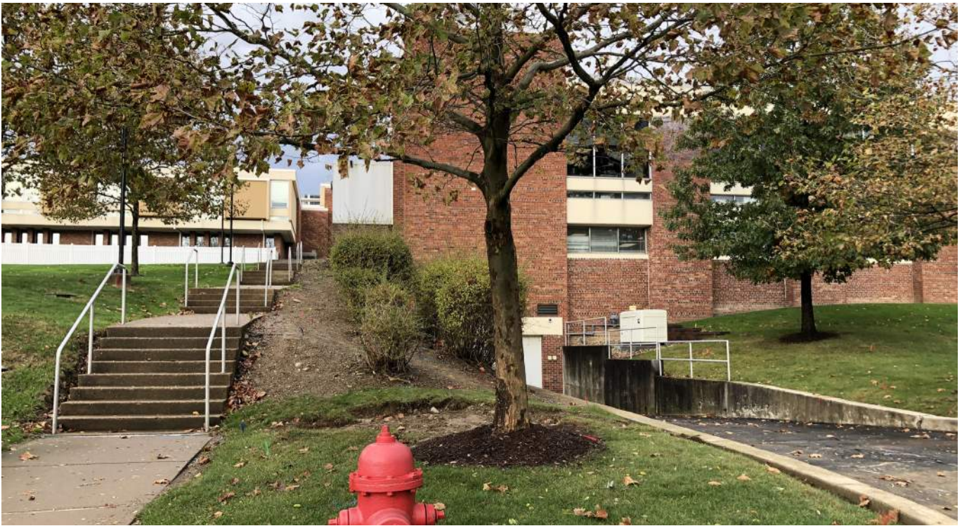
Existing Loading Dock & Adjacent Walkway
